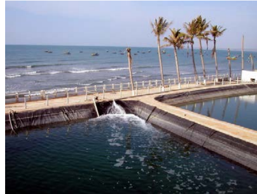
Sea water settling and filter system
