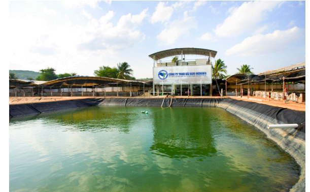
Sea water settling and filter system
